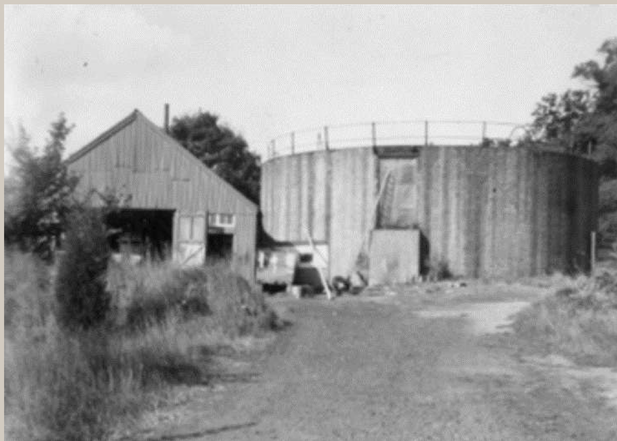
Lower diesel storage tank c. 1950
