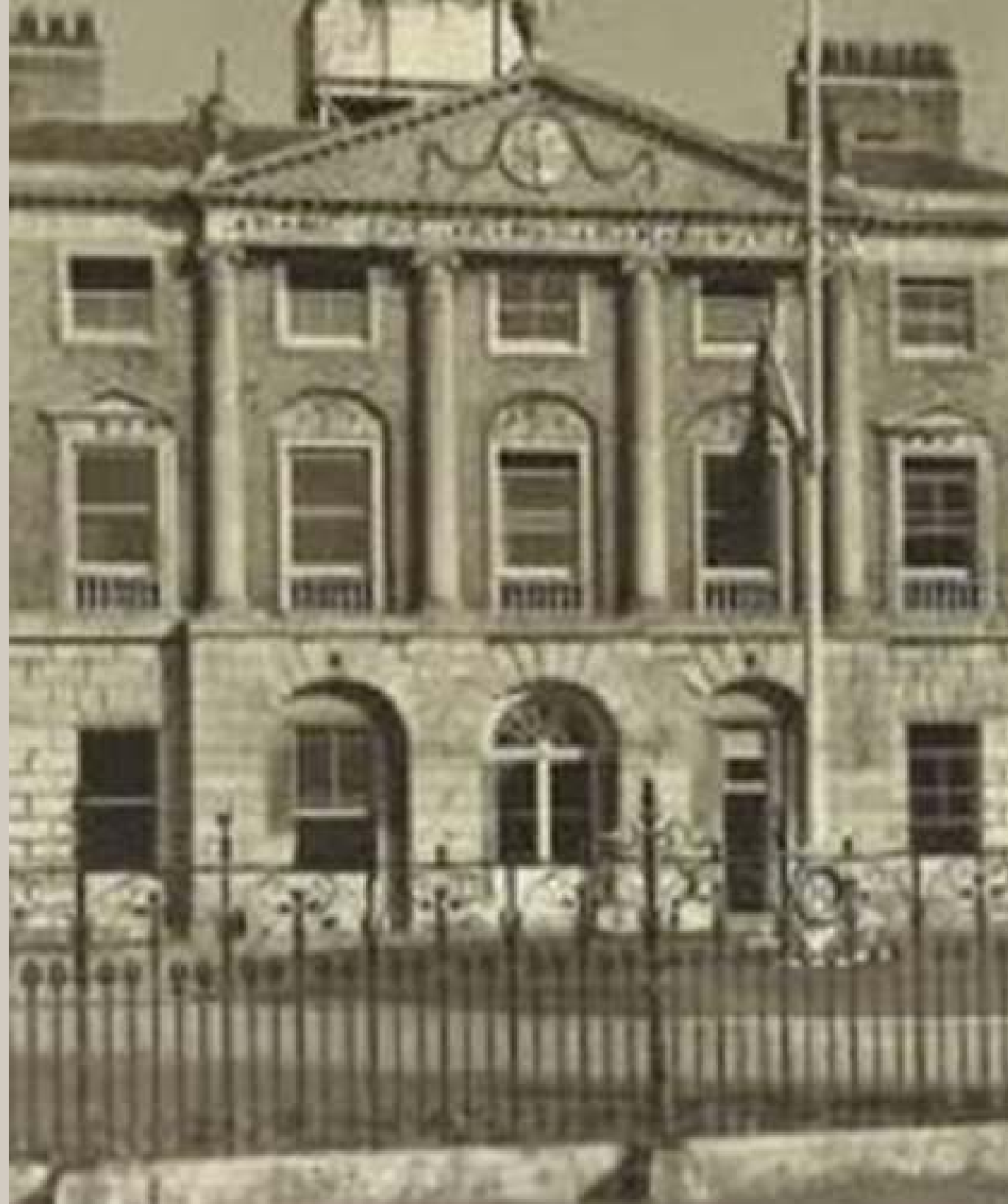
Observation staging on the roof of the Hall
